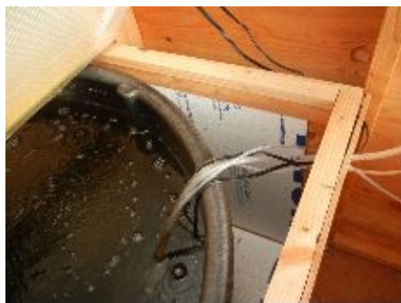
Photo 9: This is an example of installing bead board inside the fish tank to help maintain heat between 78 and 80 degrees year round . The wires go to the heaters.
