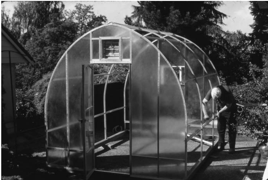
FIGURE 19.15 Assembly of gable ends, with door and exhaust shutter, to purlins. (Courtesy of Resh Greenhouses Ltd., Vancouver, British Columbia, Canada.)
